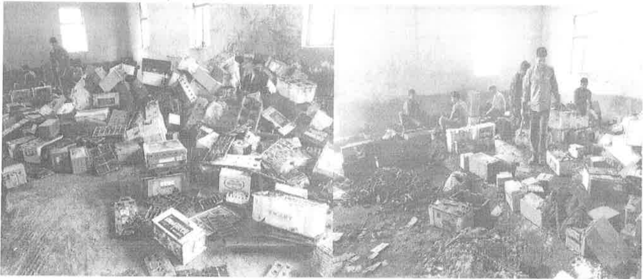
Manual Dismantling and Dump of Battery components
