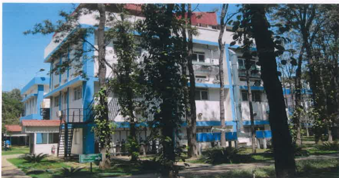
View of the plant
