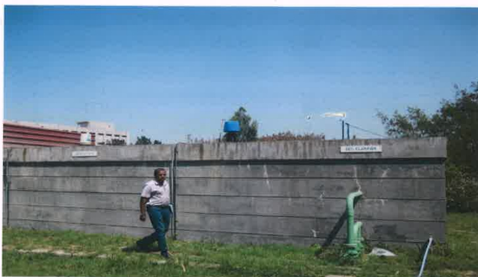
View of STP
