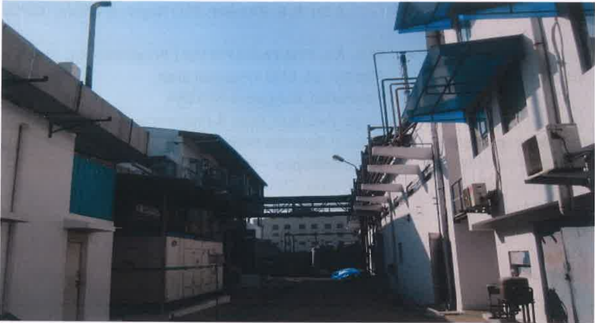
View of the Plant
