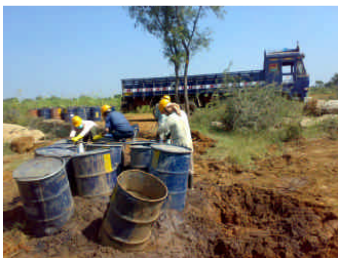
Fig. 2. Removing of waste from Koratagere dump site
